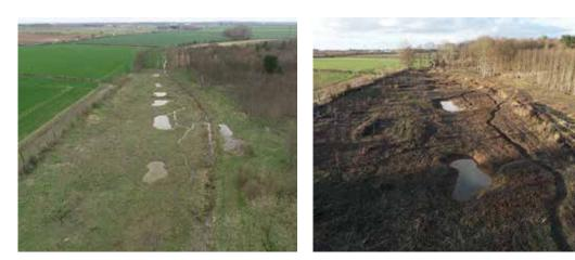
Nettleham Beck demonstration site, where a network of slightly sinuous channels and ponds were excavated to reconnect stream and floodplain. When water levels are higher wood jams in the main straightened channel force water to flow out over the floodplain (left), while the channels remain dry during periods of low flow (right). Luca Mao/University of Lincoln
