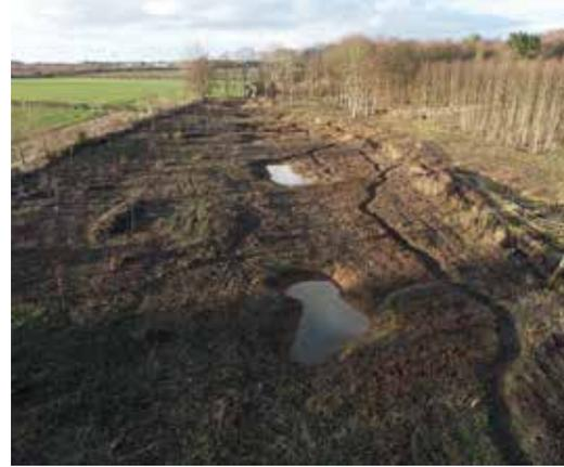
Nettleham Beck demonstration site, where a network of slightly sinuous channels and ponds were excavated to reconnect stream and floodplain. When water levels are higher wood jams in the main straightened channel force water to flow out over the floodplain (left), while the channels remain dry during periods of low flow (right). Luca Mao/University of Lincoln
